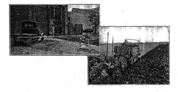
time. Far from damaging the tow paths, which is the case with so many tractors, the Citroën Kégresse tends rather to improve than to damage. The above factors, accompanied with the low running and maintenance costs of the Citroën Kégresse vehicle, makes these machines far more economical than horses for this type of traction.
